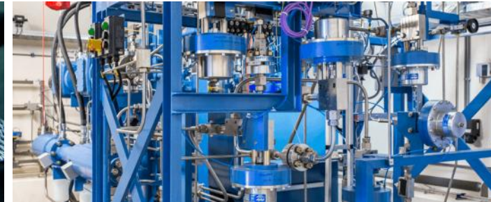
Gas Testing Laboratory
